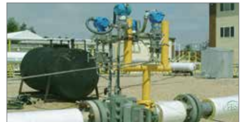
Wet Gas DPro-Orifice System
